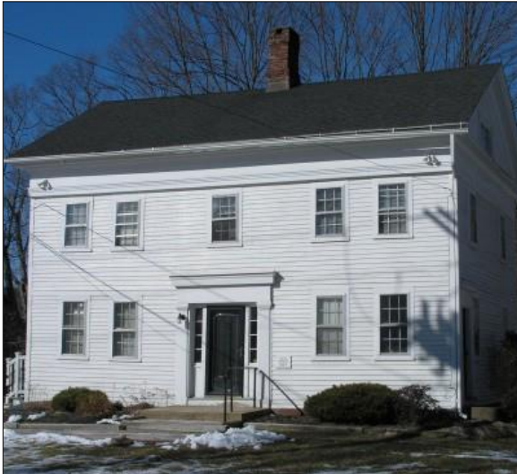
Simple, yet well detailed, wood siding
