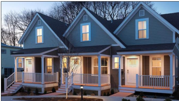
Attached single family cottages
